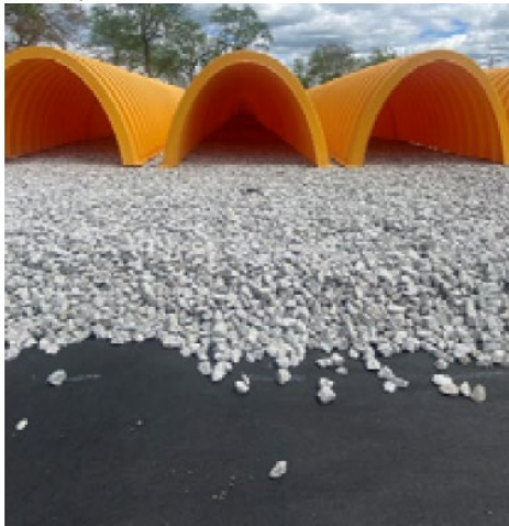
Photo #2: Close up of Chamber System Unit, Stone, and Filter Fabric . (Looking East)
