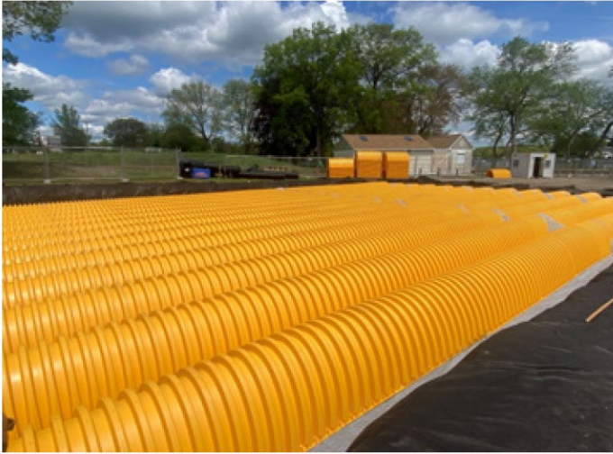
Photo #1: SC-800 Chamber System Installation Progress . (Looking North East)
