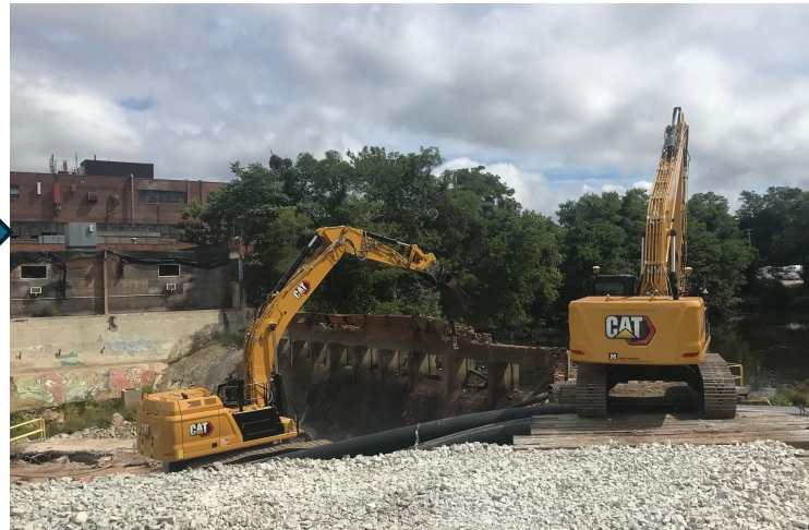
First "bites" out of the Armstrong Dam, 8/2023
