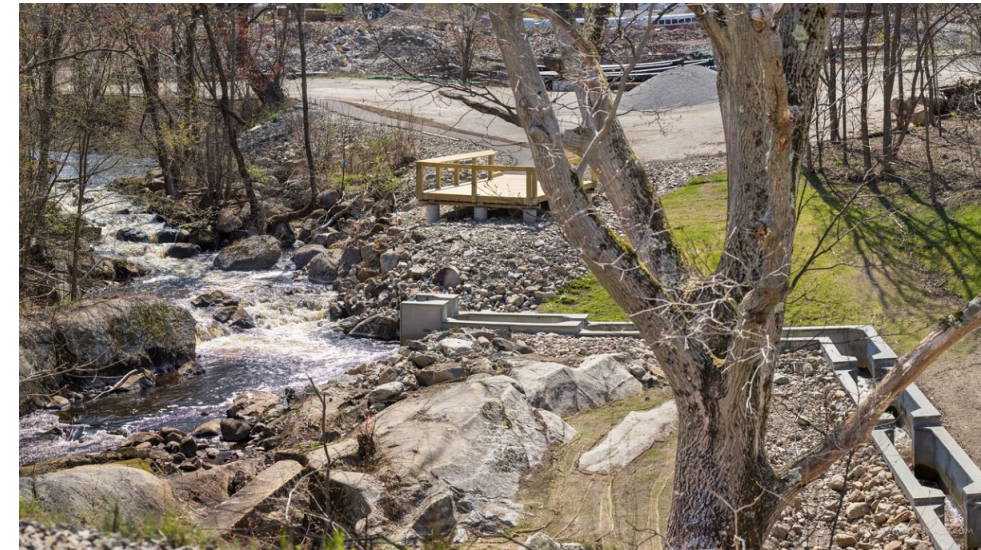
fish bypass and viewing platform
