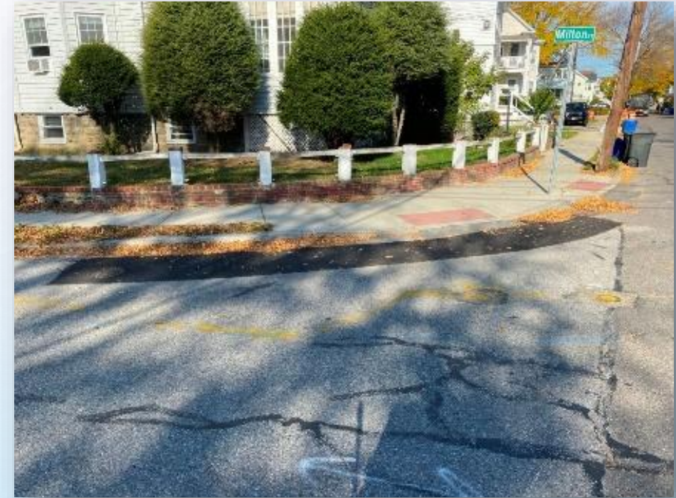
Post-construction of infiltration trench in Arlington (City of Arlington)
