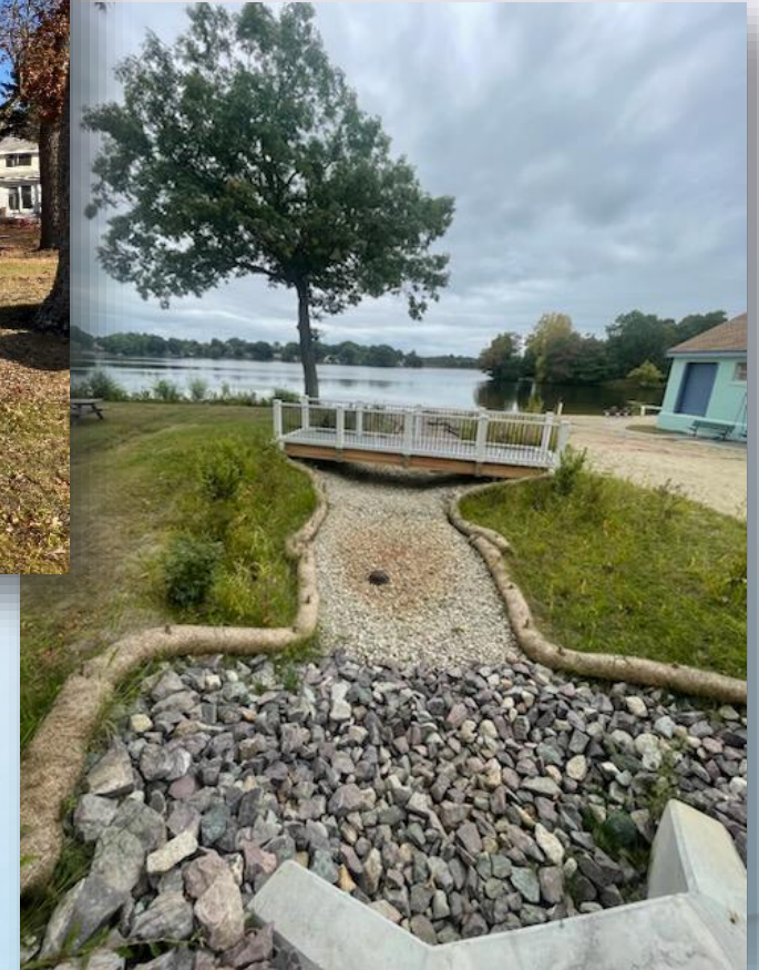
Water quality/bioretention swale installed at Lake Waushakum (City of Framingham)
