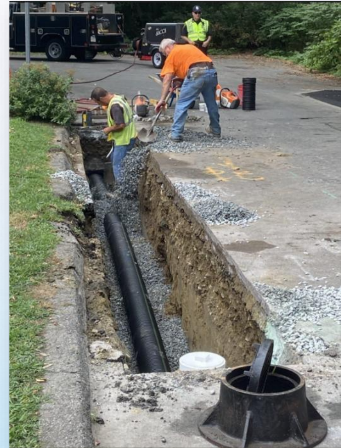
Infiltration trench being installed in the Mystic River watershed (MyRWA)
