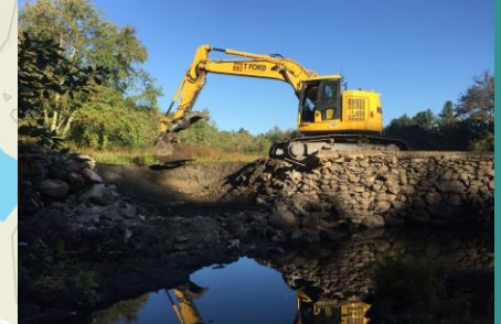
Turner Dam Removal (2015)
