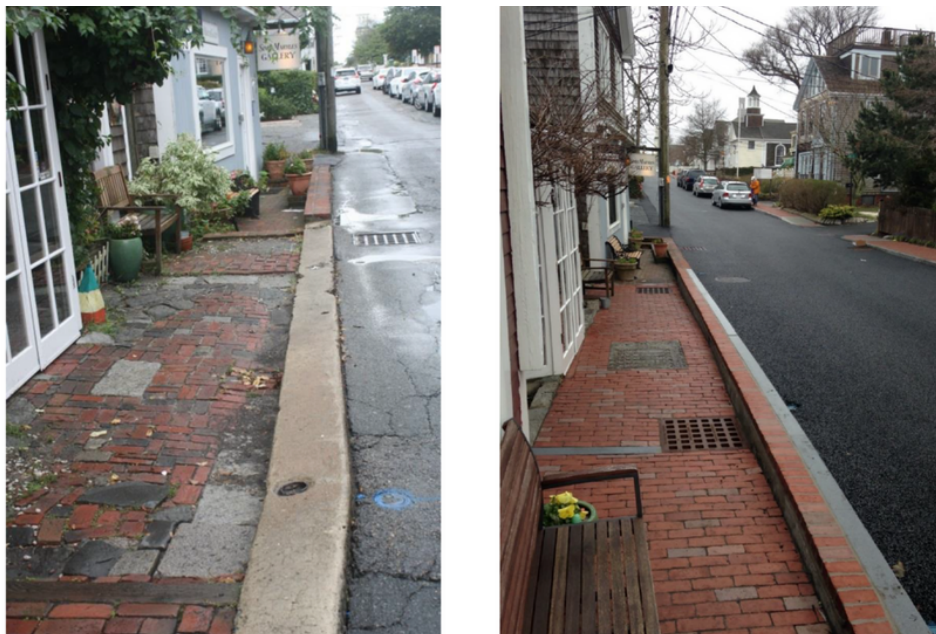
Figure 4. Image depicting the before and after of the Commercial Street Rehabilitation project in Provincetown. Source: “Provincetown Stormwater Program Revitalizes Downtown and Improves Beach Water Quality using Porous Asphalt,” Soak Up the Rain New England Webinar Series, EPA. July 28, 2020.
